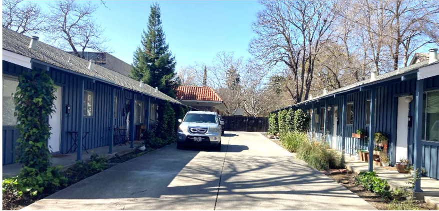
Driveway between 113 (left) and 117 C Street (right), view facing west. Source: ESA, 2024.
