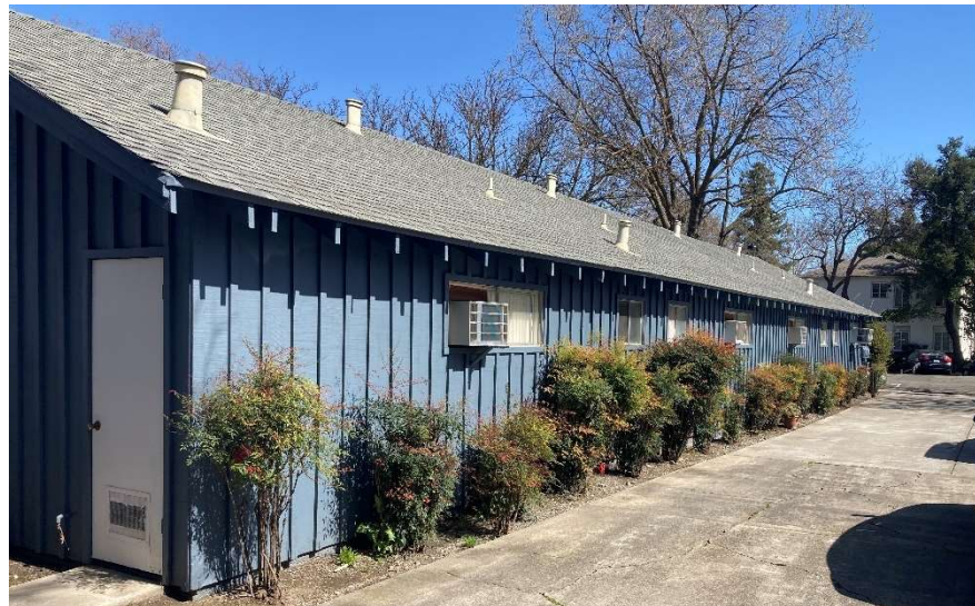
Typical rear (east-west) façade of 113 C Street, facing east. Source: ESA, 2024.
